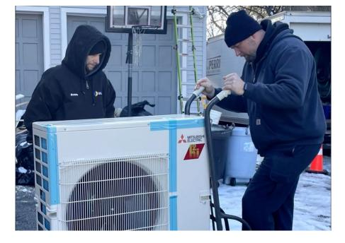
In addition to delivering comfort to rooms that need it, without installing ductwork, the system offers powerful heating even in chilly N.J. winters. Mitsubishi Electric's hyper-heating inverter technology provides 100% heating capacity down to -5° F and guaranteed operation down to -13° F.
